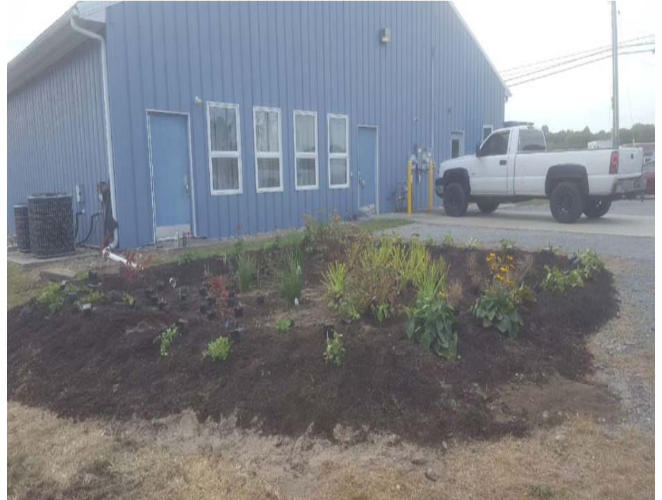
After, Rain Garden, 30 Broad Street, Elmer, NJ
